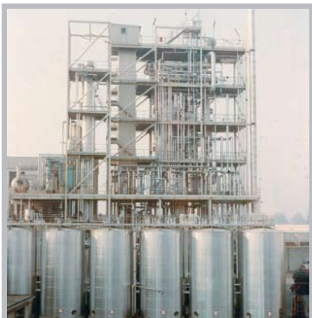
"UNITOWER" fats splitting and distillation plant Capacity: 100 t/d
