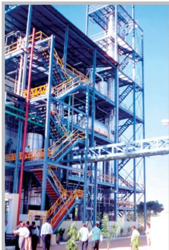
“UNITOWER” continuous fats splitting plant Capacity: 120 t/d
